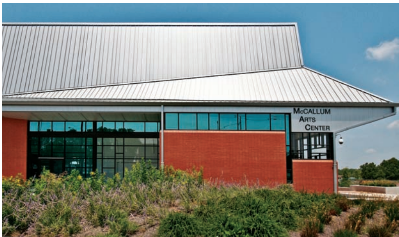
McAllum High School Fine Arts Academy draws students from across Texas' Austin Independent School District and provides an accelerated, comprehensive arts curriculum. A total of 2136 m 2 (23,000 sf) of the metal roofing panels were installed and finished in silver metallic for minimal maintenance.
