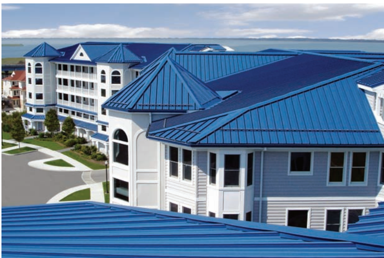
The Tides at Seaboard Point in New Jersey offers resort-style, oceanfront, multi-family living. To withstand the coastal climate conditions, PVDF resin-based coatings were used to enhance the metal roofs' corrosion-resistance and structural integrity.
