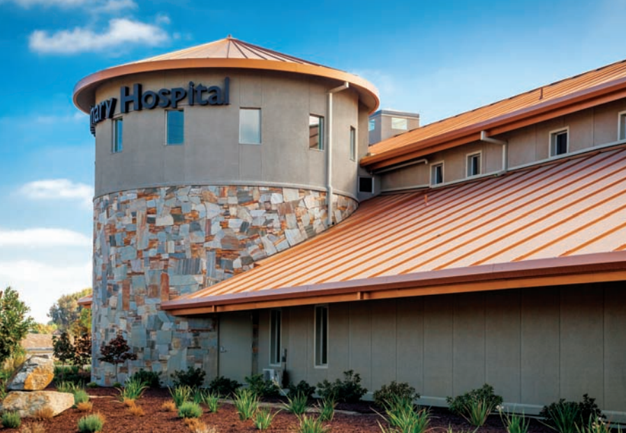
Located in Modesto, California, Beckwith Veterinary Hospital's 1300-m 2 (14,000-sf) facility used green building strategies to save resources and promote sustainability. Design features include photovoltaic (PV) power and insulated standing-seam metal roof panels with a copper finish.
