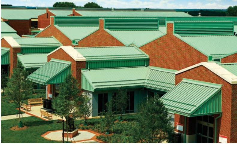
To create the distinctive metal roof on the 10,219-m 2 (110,000-sf) Randall B. Terry, Jr. Companion Animal Veterinary Center at North Carolina State University in Raleigh, a three-coat system in a custom color with a clear coat was specified.
