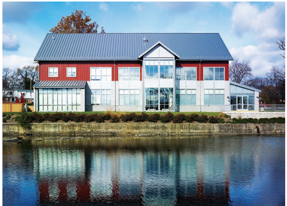
Located under the metal roof of Davis Hall, Shenandoah University's History and Tourism Center in Winchester, Virginia, features metal roofing panels, finished in a 70 percent PVDF coating system.
