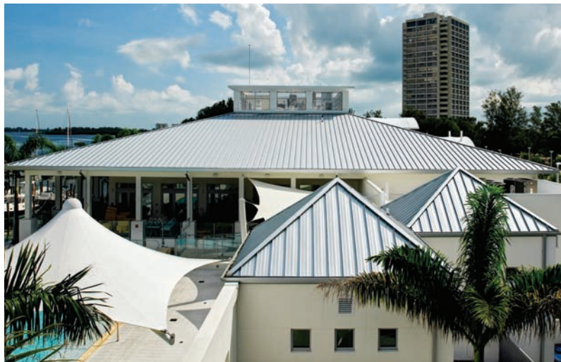
The metal roof on Florida's 2136-m 2 (23,000-sf) Sarasota Yacht Club was built to meet the stringent Florida Building Code (FBC) using aluminum panels. The 406-mm (16-in.) wide aluminum panels were finished in silver with a 70 percent polyvinylidene fluoride (PVDF) resin-based coating that withstands extended exterior exposure to water, humidity, temperature, ultraviolet (UV) light, and oxygen, along with atmospheric pollutants.
